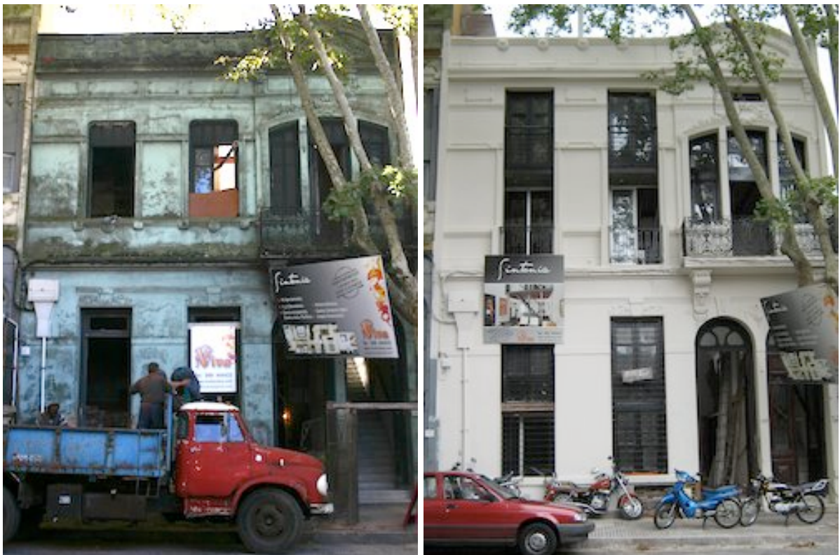
THE FACADE, BEFORE AND AFTER
